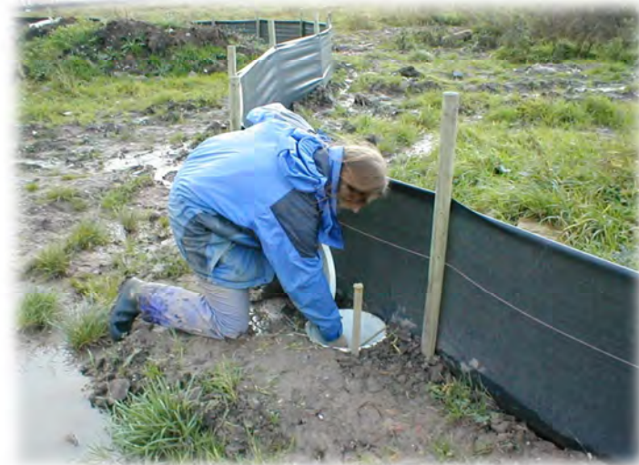
Figure 3: Newt exclusion fencing and capture of newts from development sites within 500m of a breeding GCN pond prior to development commencing is a common mitigation measure.
